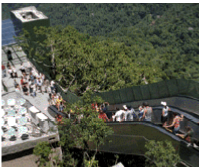
Tourists riding the escalator down toward the elevators. The Gen2 hoistway is at top left.
